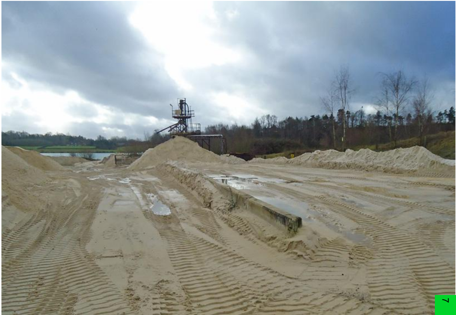
Figure 1 : View south previous plant and stockpiles at northern end of site
