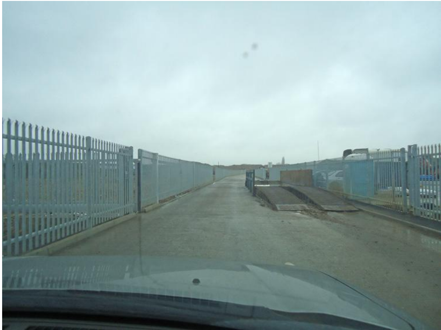
Figure 3 : View of existing internal access haul road facing west
